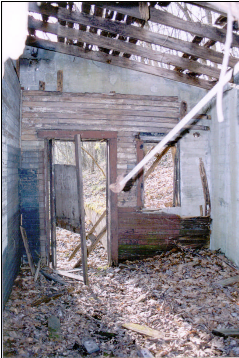
Figure 38. Interior view of the second addition to the fan house, looking west. This room is believed to have served as an office. Note the wainscoting applied to the walls (FRR April 2003).
