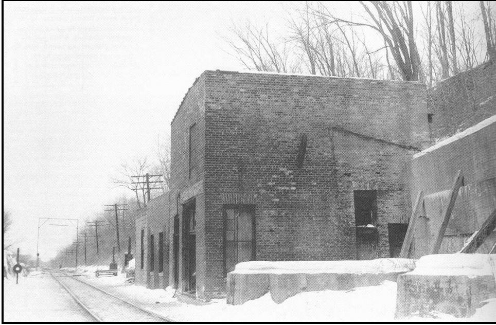
Figure 22. Another view of the fan house complex in 1961, looking northwest. The concrete foundations and failing retaining wall in the foreground mark the former location of the ventilation fan (Huddleston 1998:56)
