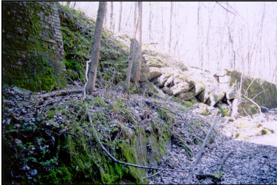
Figure 40. The dry-laid masonry wall constructed as a part of the 1902 tunnel renovation largely remains intact along the south side of the rail bed, opposite from the fan house. It is a contributing feature to the site (FRR April 2003).
