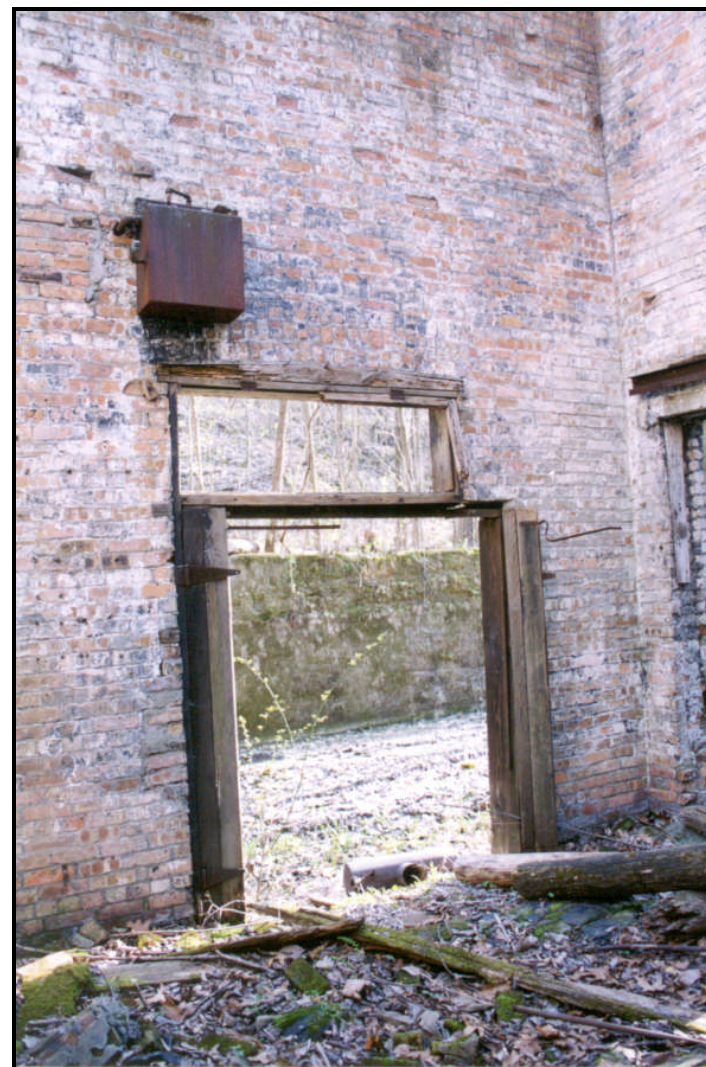
Figure 32. Exterior (LEFT) and interior (RIGHT) views of the original entrance to the engine room. This doorway was widened early in the twentieth century. Note the fanlight above the door (FRR April 2003).
