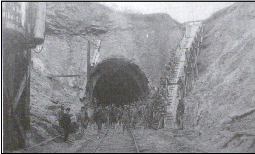
Figure 6. Photograph of the east portal to the Winston Tunnel during the 1902 renovation. The brick-and-concrete facing on the portal had yet to be built (Huddleston 1998:42).
