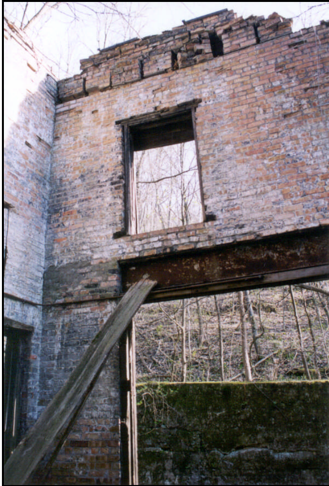
Figure 33. (LEFT) The wide freight door and upper-level window shown here represent modifications to the engine room. (RIGHT) View of the northwest corner of the engine room, showing the large (fuel?) tanks located here. The engine has been removed (FRR April 2003).
