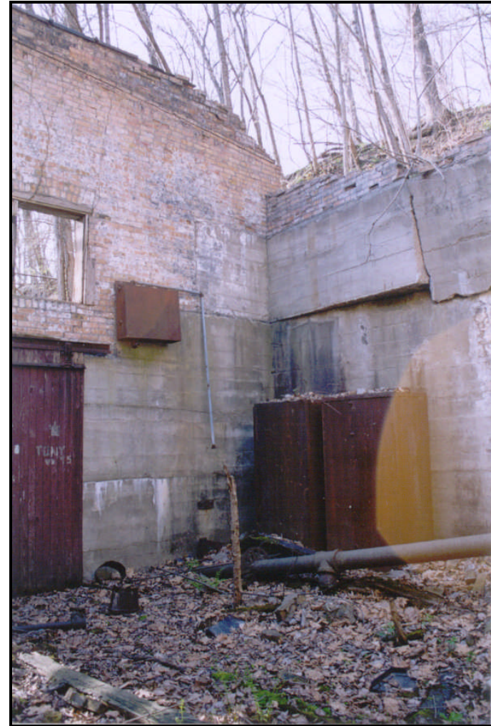
Figure 33. (LEFT) The wide freight door and upper-level window shown here represent modifications to the engine room. (RIGHT) View of the northwest corner of the engine room, showing the large (fuel?) tanks located here. The engine has been removed (FRR April 2003).
