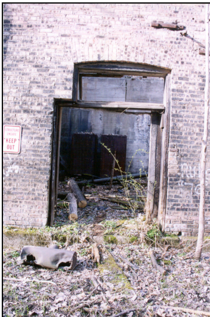
Figure 32. Exterior (LEFT) and interior (RIGHT) views of the original entrance to the engine room. This doorway was widened early in the twentieth century. Note the fanlight above the door (FRR April 2003).
