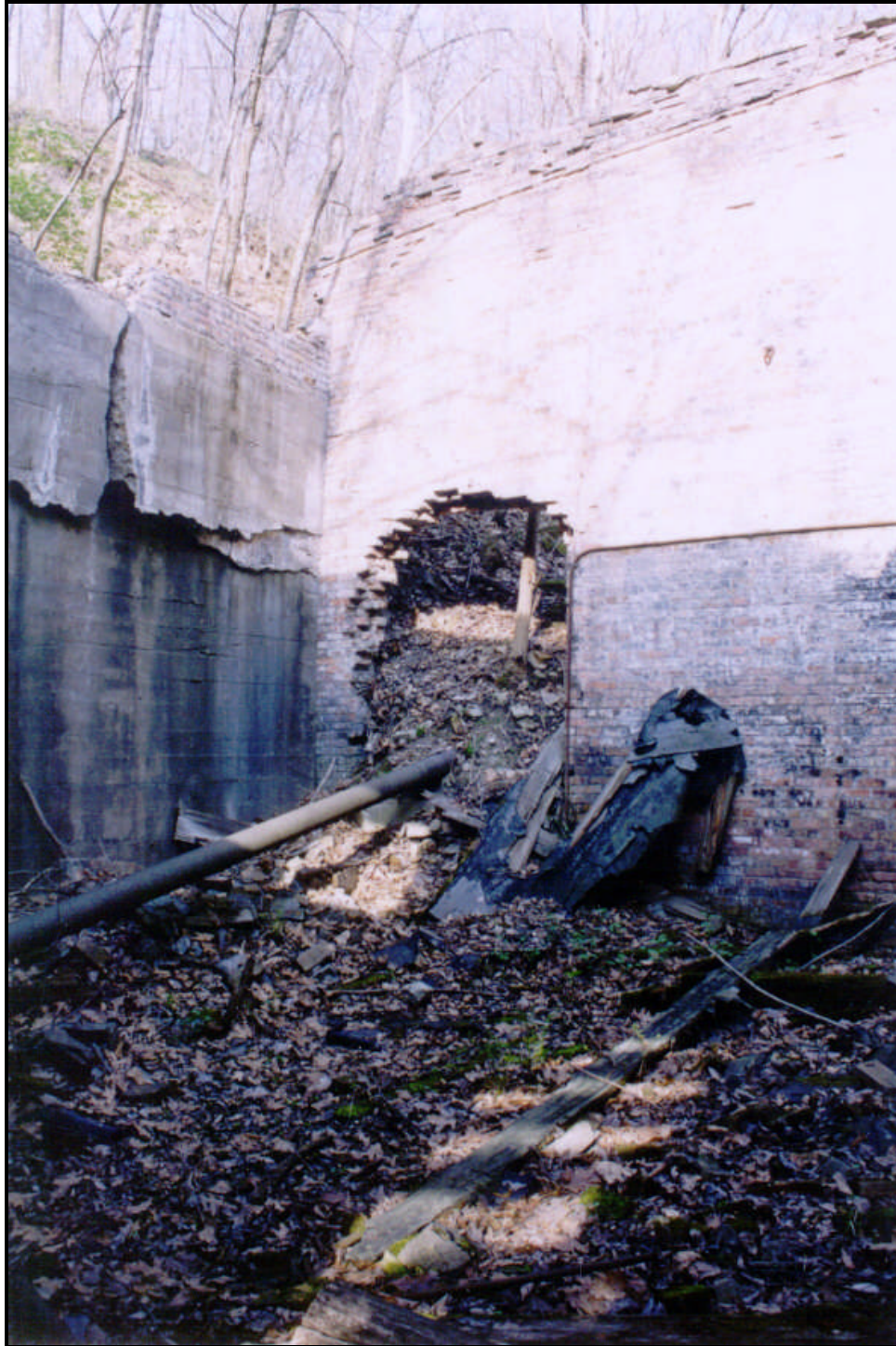
Figure 34. View of the east side of the engine room, showing the collapsed section of wall where the fan belt formerly passed through. The function of the large pipe lying across the room is not known (FRR April 2003).
