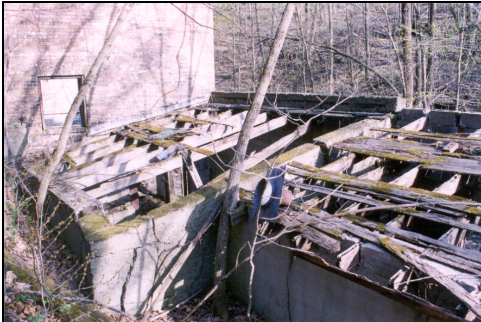
Figure 39. The fan house has suffered from both vandalism and decay since its abandonment in 1948. (TOP) Graffiti inscribed on the wainscoting in the office addition. (BOTTOM) View of the deteriorated roofs over the office and pump room additions (FRR April 2003).
