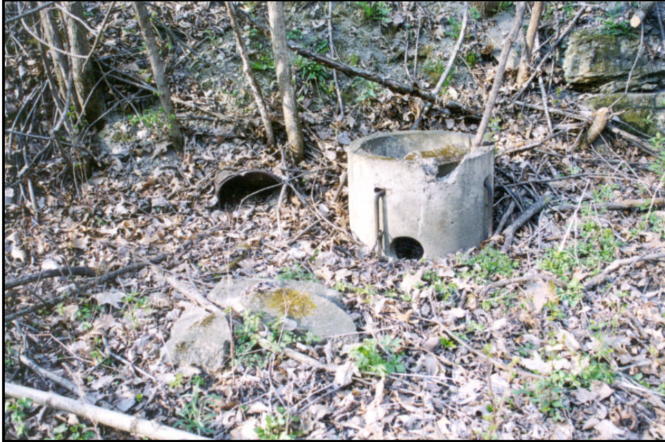
Figure 41. The top to a concrete-lined well located behind the fan-house complex (FRR April 2003).
