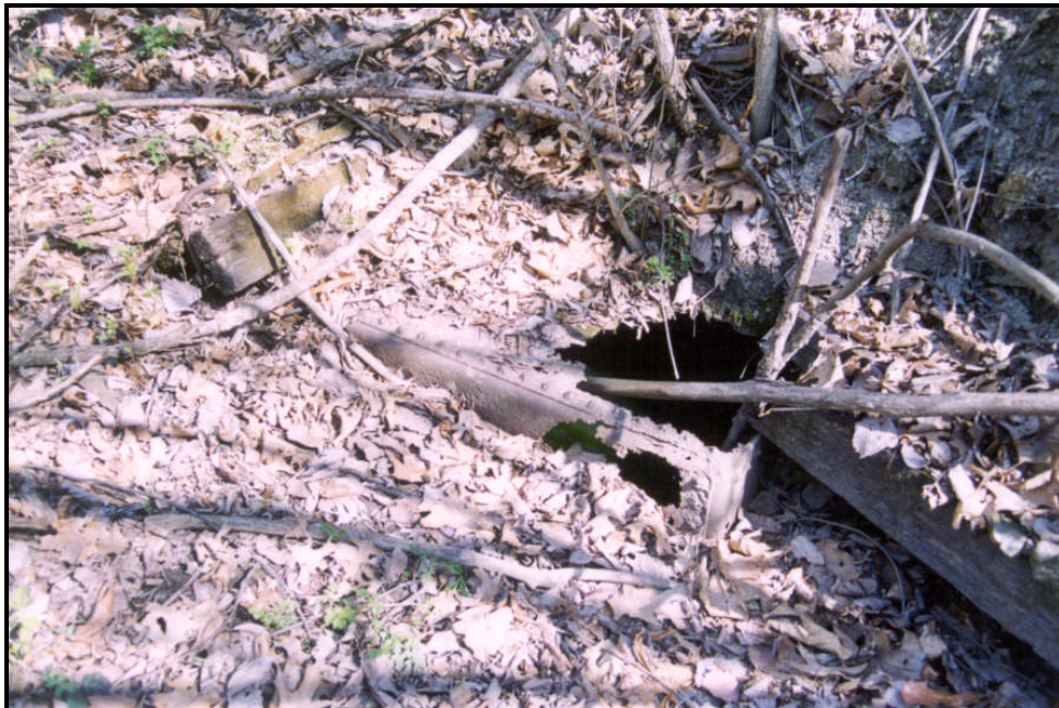
Figure 42. A steel fuel tank buried by overburden (FRR April 2003).
