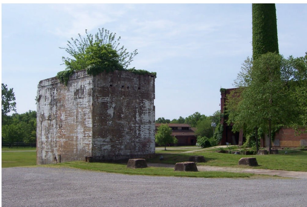
Figure 42. Two views of the concrete base for the headframe over Shaft A, looking south. The concrete piers shown at center once supported steel uprights for the screening structure (FRR May 2006).
