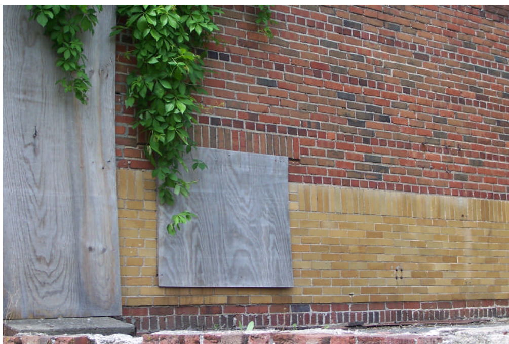
Figure 28. Detail of the common partition wall between the two rooms in the hoist engine house. Note the use of glazed brick, as a kind of wainscoting, on the lower portion of the wall. A similar treatment was employed in the powerhouse. The plywood panels cover a doorway and window opening (FRR May 2006).
