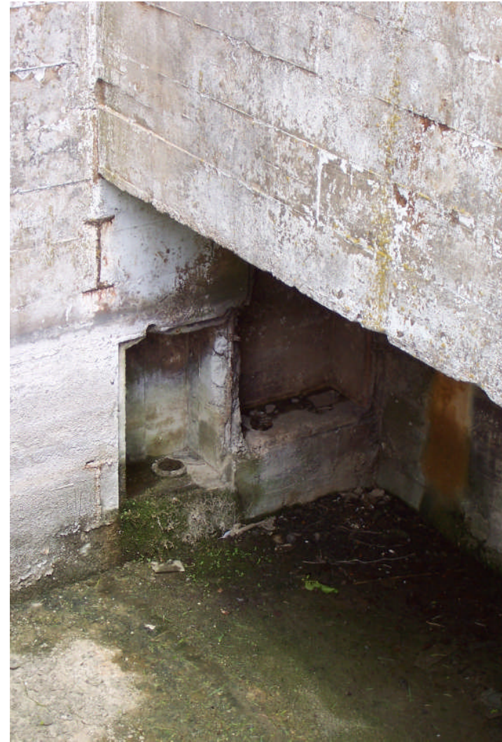
Figure 40. Views looking down into Shaft A, which is sealed off with a 16"-thick concrete cap approximately 8' below the ground surface. (LEFT) The steel ladder leading down to the cap level. (RIGHT) View of two niches in the northeast corner of the shaft, which may have held electrical panels at one time (FRR May 2006).
