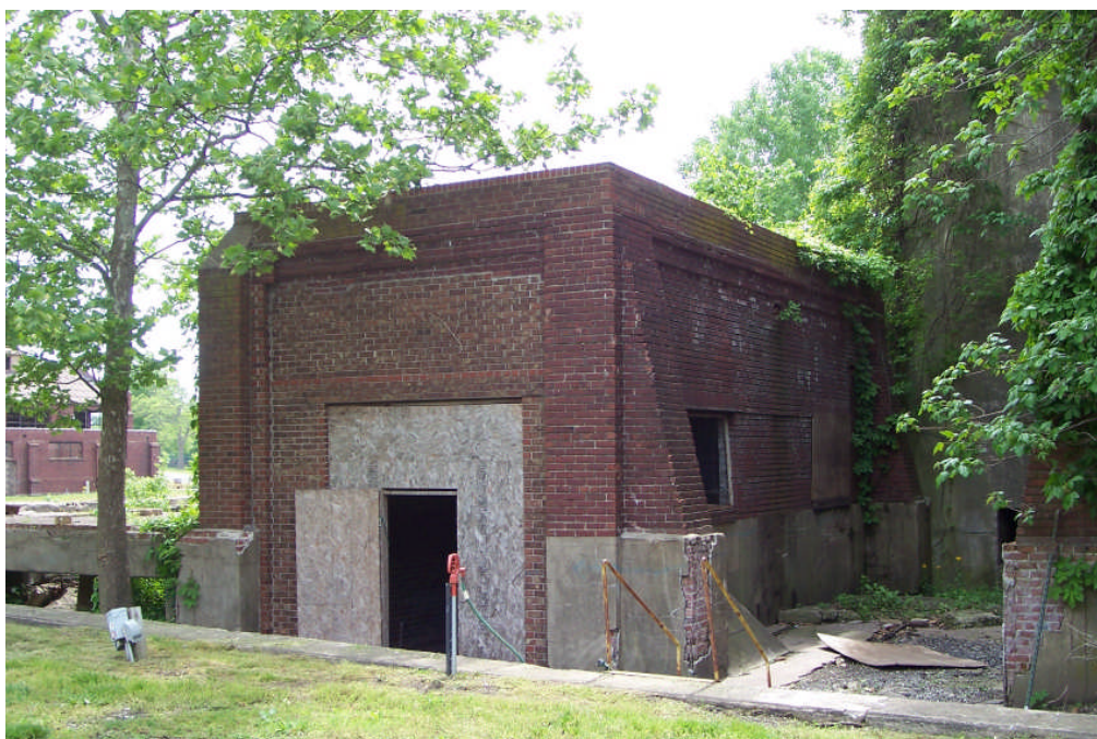
Figure 35. Exterior view of the west end of the hoist-engine house, which largely remains intact. The buttresses on the building are similar to those found on the adjacent powerhouse (FRR May 2006).
