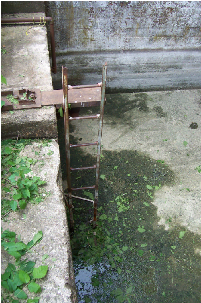
Figure 40. Views looking down into Shaft A, which is sealed off with a 16"-thick concrete cap approximately 8' below the ground surface. (LEFT) The steel ladder leading down to the cap level. (RIGHT) View of two niches in the northeast corner of the shaft, which may have held electrical panels at one time (FRR May 2006).
