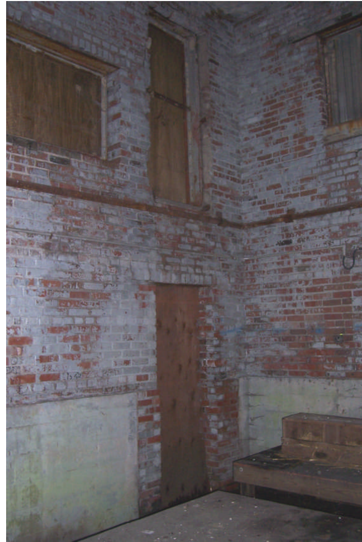
Figure 36. Interior views of the west room in the hoist-engine house. This room possibly held a regulator tank(s?) where steam produced in the adjacent powerhouse was converted for use by the hoist engine. The room had doorway accessing both the basement and main levels of the adjacent engine room (FRR May 2006).
