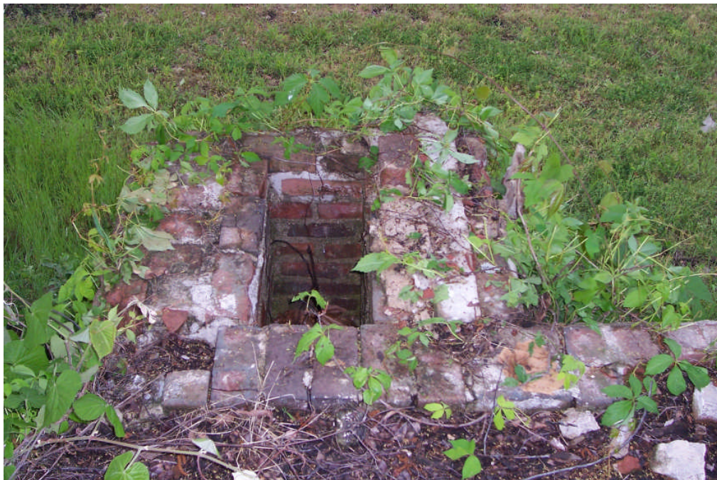
Figure 31. View of the one of the brick piers on the east end of the hoist engine house, on which the diagonal braces for the tippie over Shaft A rested (FRR May 2006).
