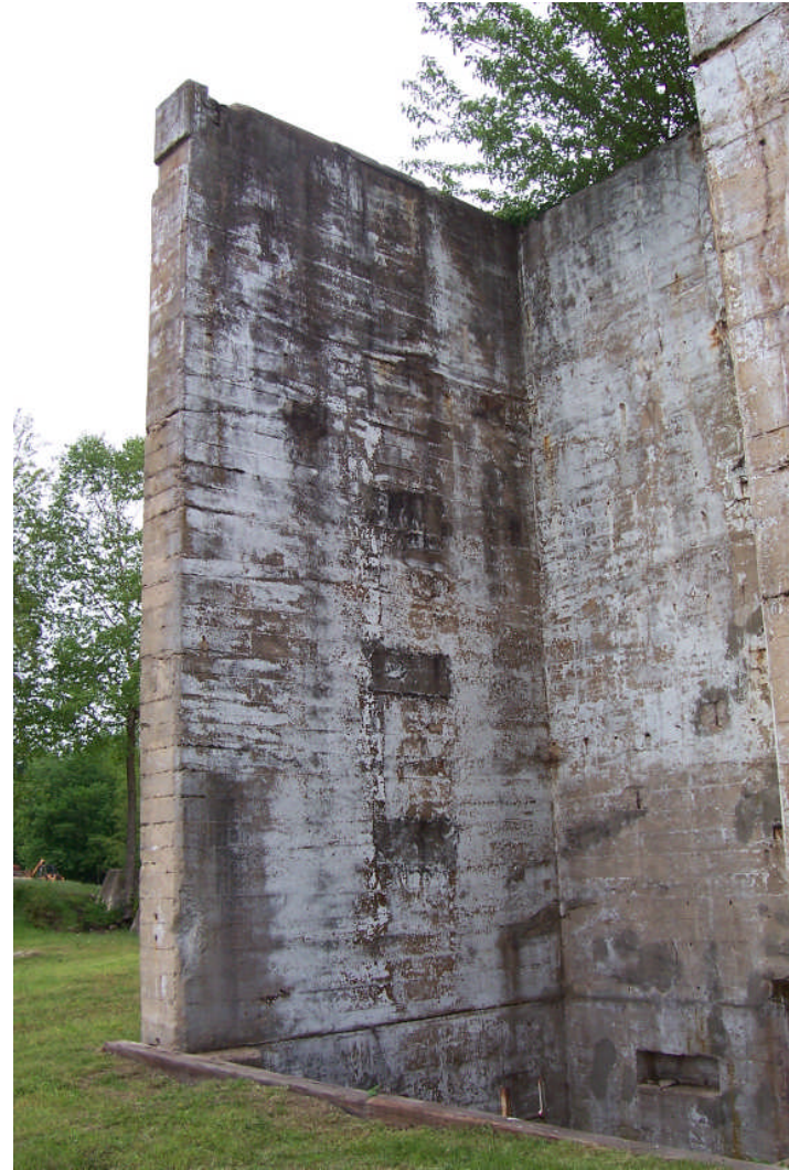
Figure 39. Two views of the concrete base for the headframe over Shaft A, showing the southern of its two “cells” where the shaft proper was located. When in operation, Shaft A employed a dual hoisting system, with two cages present. The steel framework for the hoisting mechanism has been removed (FRR May 2006).
