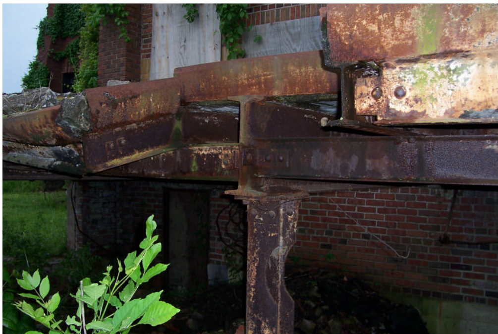
Figure 34. The main level of the hoist engine room had a reinforced-concrete floor supported by steel I-beams (FRR May 2006).
