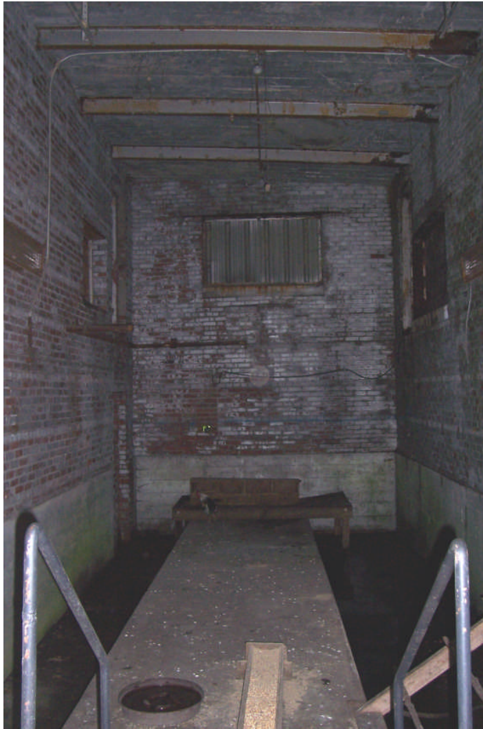
Figure 36. Interior views of the west room in the hoist-engine house. This room possibly held a regulator tank(s?) where steam produced in the adjacent powerhouse was converted for use by the hoist engine. The room had doorway accessing both the basement and main levels of the adjacent engine room (FRR May 2006).
