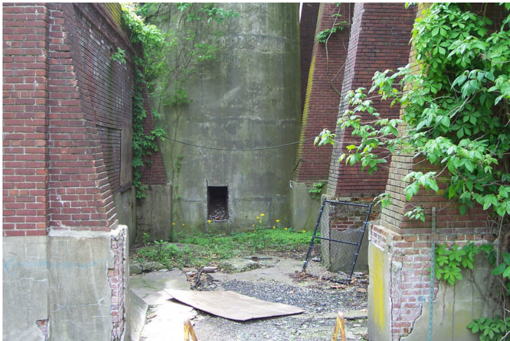
Figure 46. View of the base of the smokestack (Building/Feature 6) for the powerhouse, showing the ash cleanout on its north side. The powerhouse (Building 1) appears at right and the hoist-engine house (Building 4) for Shaft A at left (FRR May 2006).
