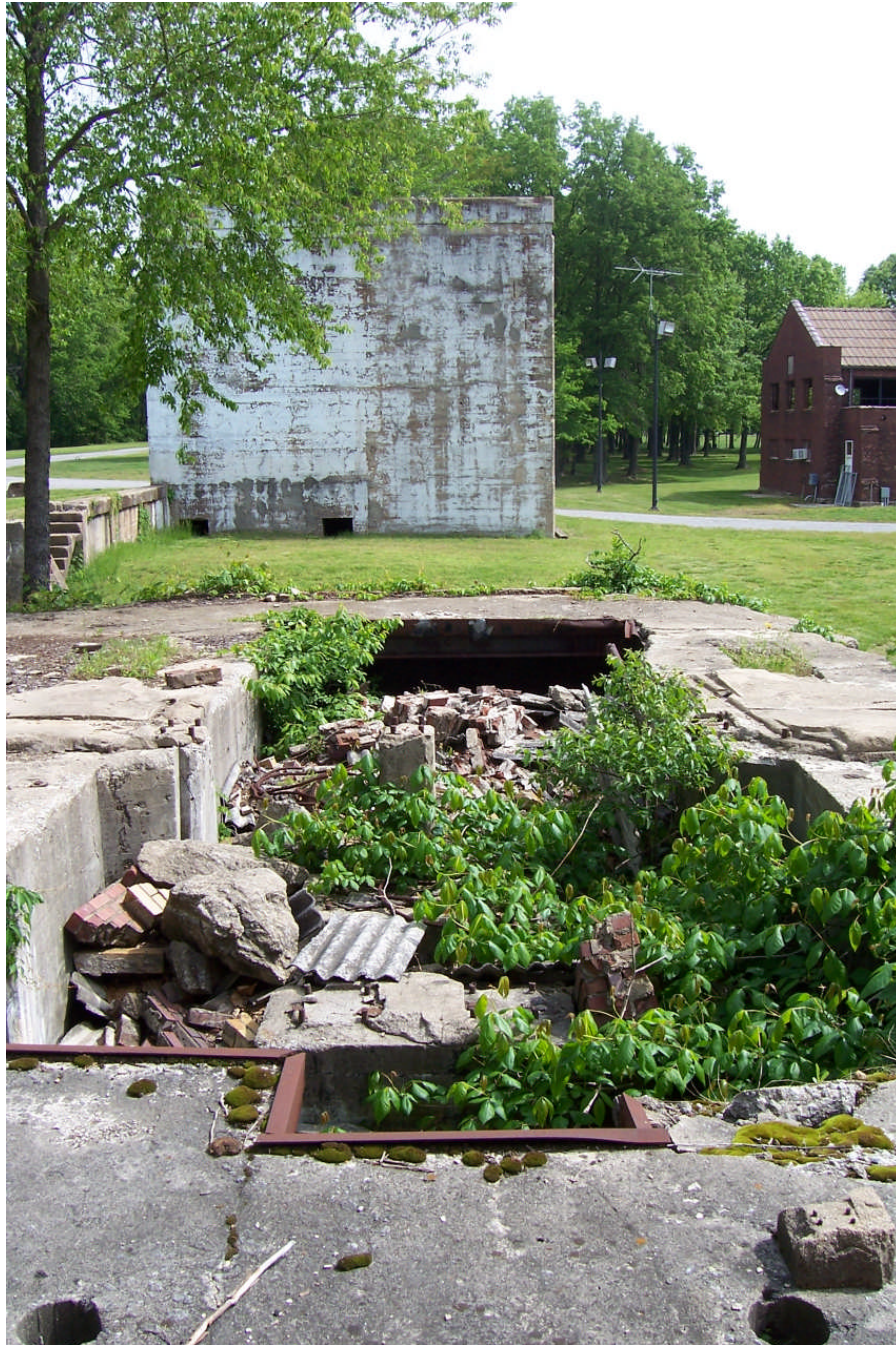
Figure 29. View looking down the length of the hoist engine room, showing the opening in the floor over which the hoist was mounted. Shaft A appears in the background (FRR May 2006).
