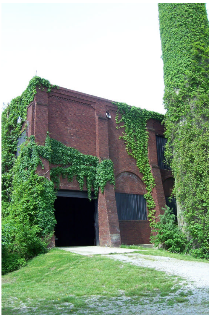
Figure 13. (LEFT) Detail of the east elevation of the powerhouse, showing the massive wall buttresses and corbelled brick cornice on the building. (RIGHT) View of the concrete storage bin on the north side of the powerhouse. This structure possibly was used to hold coal, or perhaps waste cinders, when the powerhouse was in operation. A roadway (or railway) ran beneath it (FRR May 2006).
