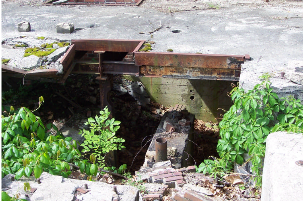
Figure 30. View looking into the basement beneath the hoist-engine room, showing one of the footings and a steam pipe for the hoist (FRR May 2006).
