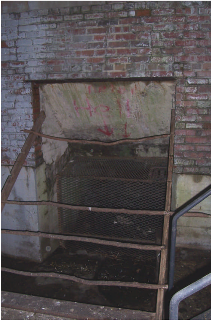
Figure 37. (LEFT) Interior view of the underground utility chase running between the hoist-engine room and powerhouse. This chase possibly was utilized to run steam pipes originally. (RIGHT) Exterior view of the west side of the hoist-engine room, showing the location of the utility chase (with sloped concrete roof) (FRR May 2006).
