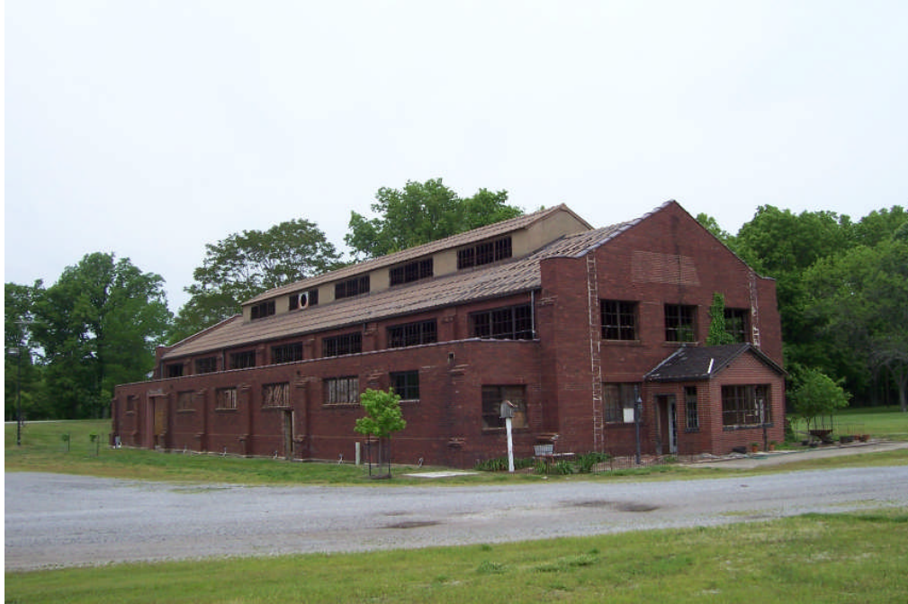
Figure 15. Exterior view of the wash house (Building 2) at the Jefferson No. 20 Mine, looking north. Despite this building's very utilitarian purpose, considerable attention was paid to its aesthetic appeal, as evidenced by the faux buttresses, stepped gable end walls, and tile roof (FRR May 2006).
