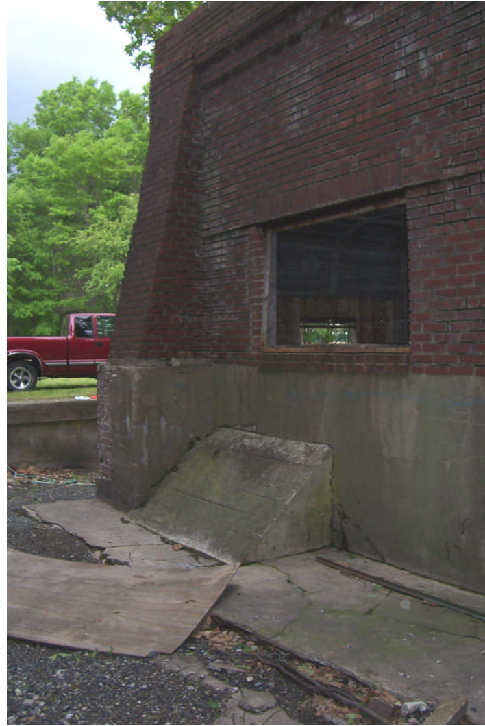
Figure 37. (LEFT) Interior view of the underground utility chase running between the hoist-engine room and powerhouse. This chase possibly was utilized to run steam pipes originally. (RIGHT) Exterior view of the west side of the hoist-engine room, showing the location of the utility chase (with sloped concrete roof) (FRR May 2006).
