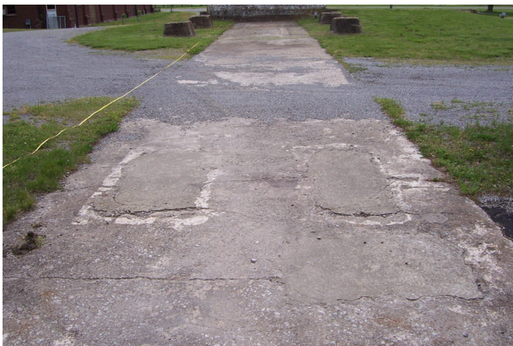
Figure 43. A concrete-lined, underground corridor runs the length of the demolished tipple structure. The roof of this corridor is exposed at grade, as shown above (FRR May 2006).
