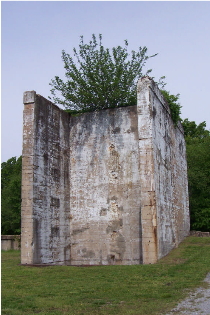
Figure 39. Two views of the concrete base for the headframe over Shaft A, showing the southern of its two “cells” where the shaft proper was located. When in operation, Shaft A employed a dual hoisting system, with two cages present. The steel framework for the hoisting mechanism has been removed (FRR May 2006).
