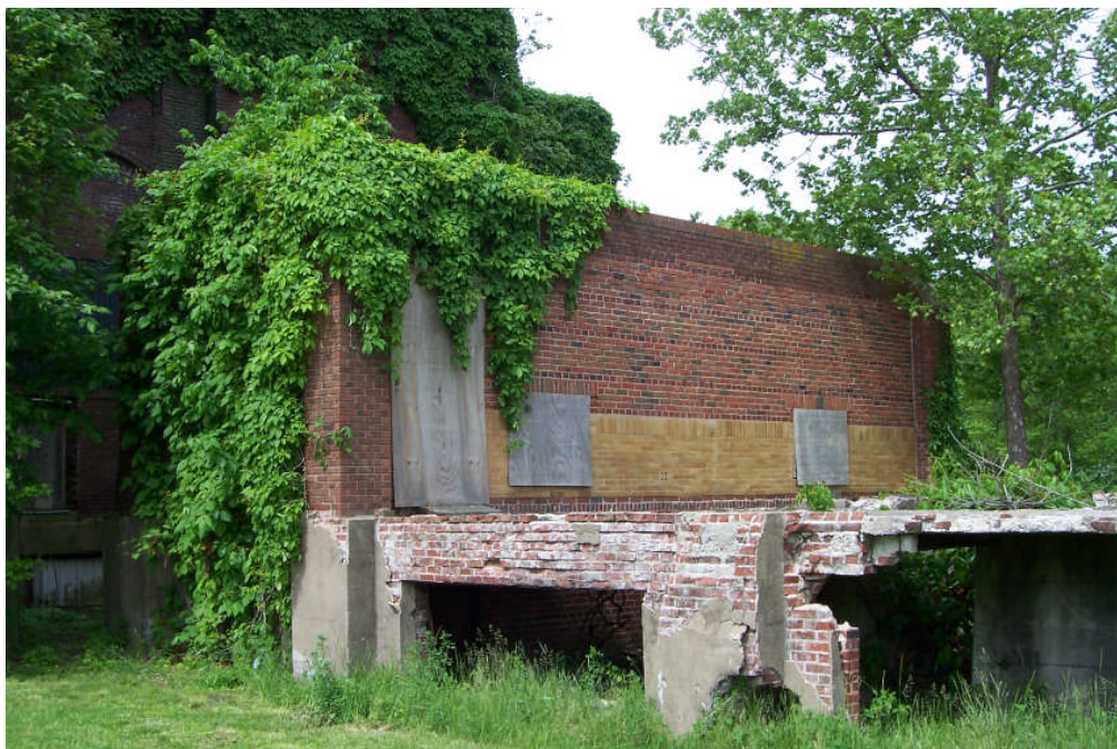
Figure 27. View of the south side of the hoist engine house for Shaft A. The west room of the building (at left) remains intact, while the larger east room (in which the hoist engine was located) has been demolished down to the foundations (FRR May 2006).
