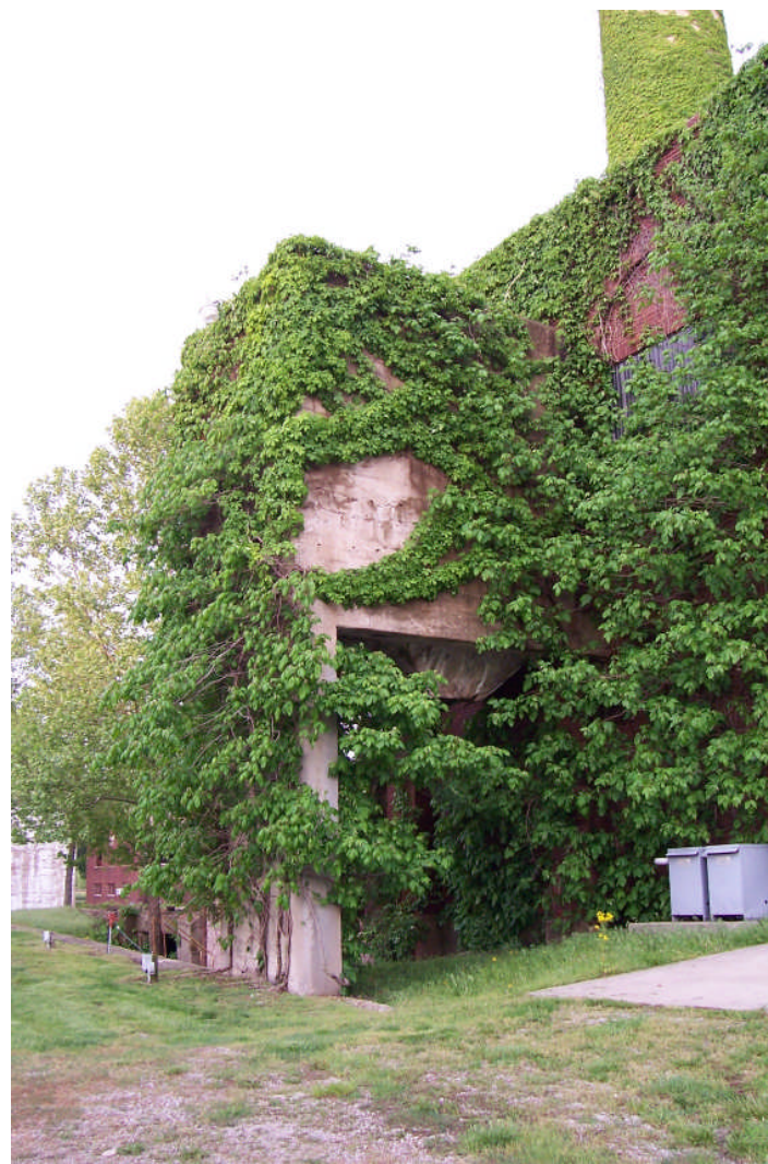
Figure 13. (LEFT) Detail of the east elevation of the powerhouse, showing the massive wall buttresses and corbelled brick cornice on the building. (RIGHT) View of the concrete storage bin on the north side of the powerhouse. This structure possibly was used to hold coal, or perhaps waste cinders, when the powerhouse was in operation. A roadway (or railway) ran beneath it (FRR May 2006).
