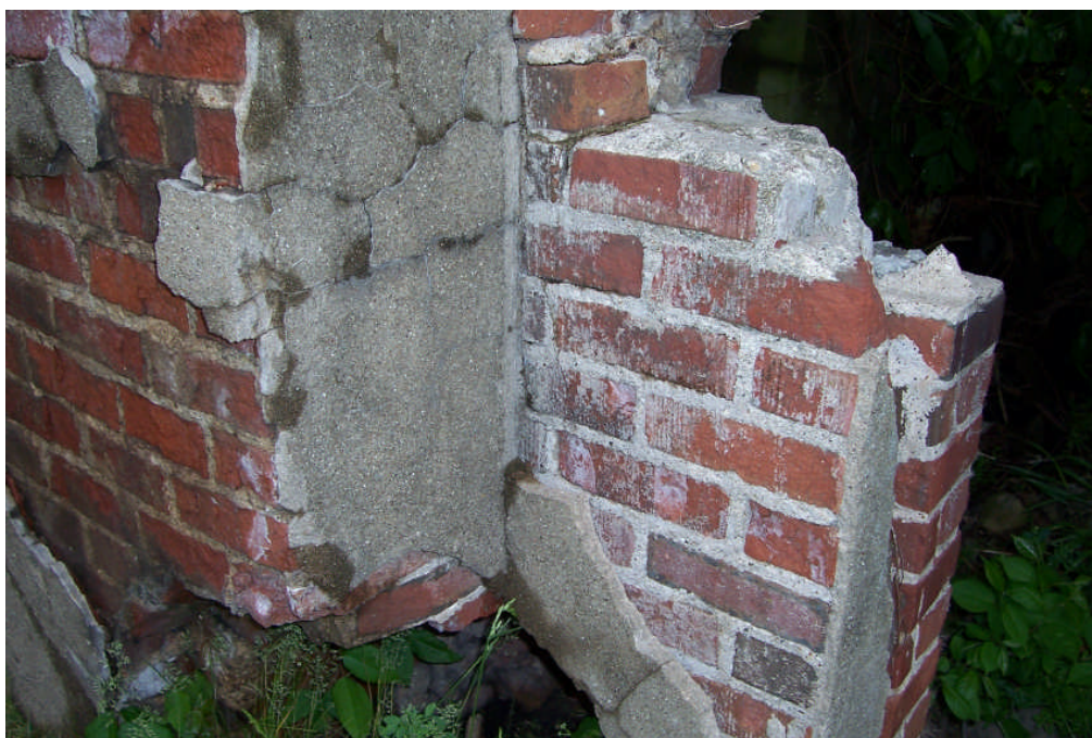
Figure 33. Detail of the foundations of the hoist engine house, showing the character of construction. The foundations were brick, set on concrete footings, and their exterior face was parged with mortar (FRR May 2006).
