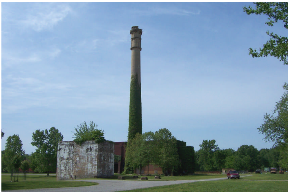
Figure 11. View of the central area of the mine site, looking south, showing concrete-lining for Shaft A (at left), the hoist-engine house remains, the powerhouse, and associated smokestack. The proposed mine reclamation work with focus on this area (FRR May 2006).
