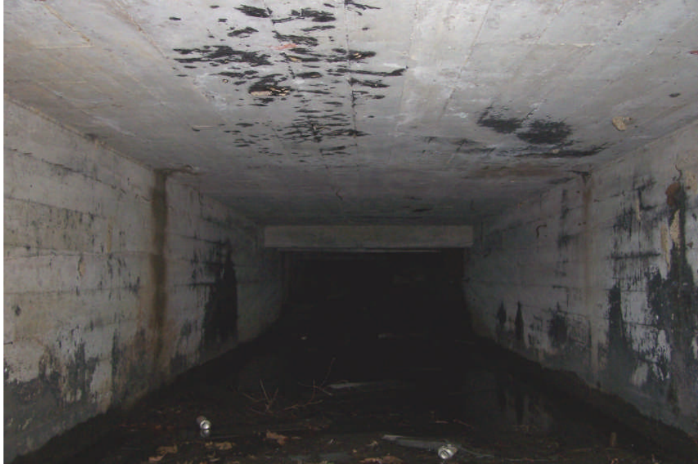
Figure 45. Interior view of the corridor beneath the tipple complex. This feature may have served a utility corridor, such as for pipes draining water out of the mine or perhaps for conveyors moving mine waste (FRR May 2006).
