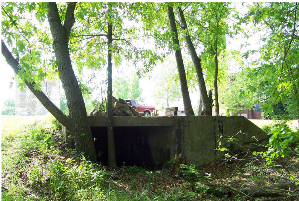
Figure 43. A concrete-lined, underground corridor runs the length of the demolished tipple structure. The roof of this corridor is exposed at grade, as shown above (FRR May 2006).
