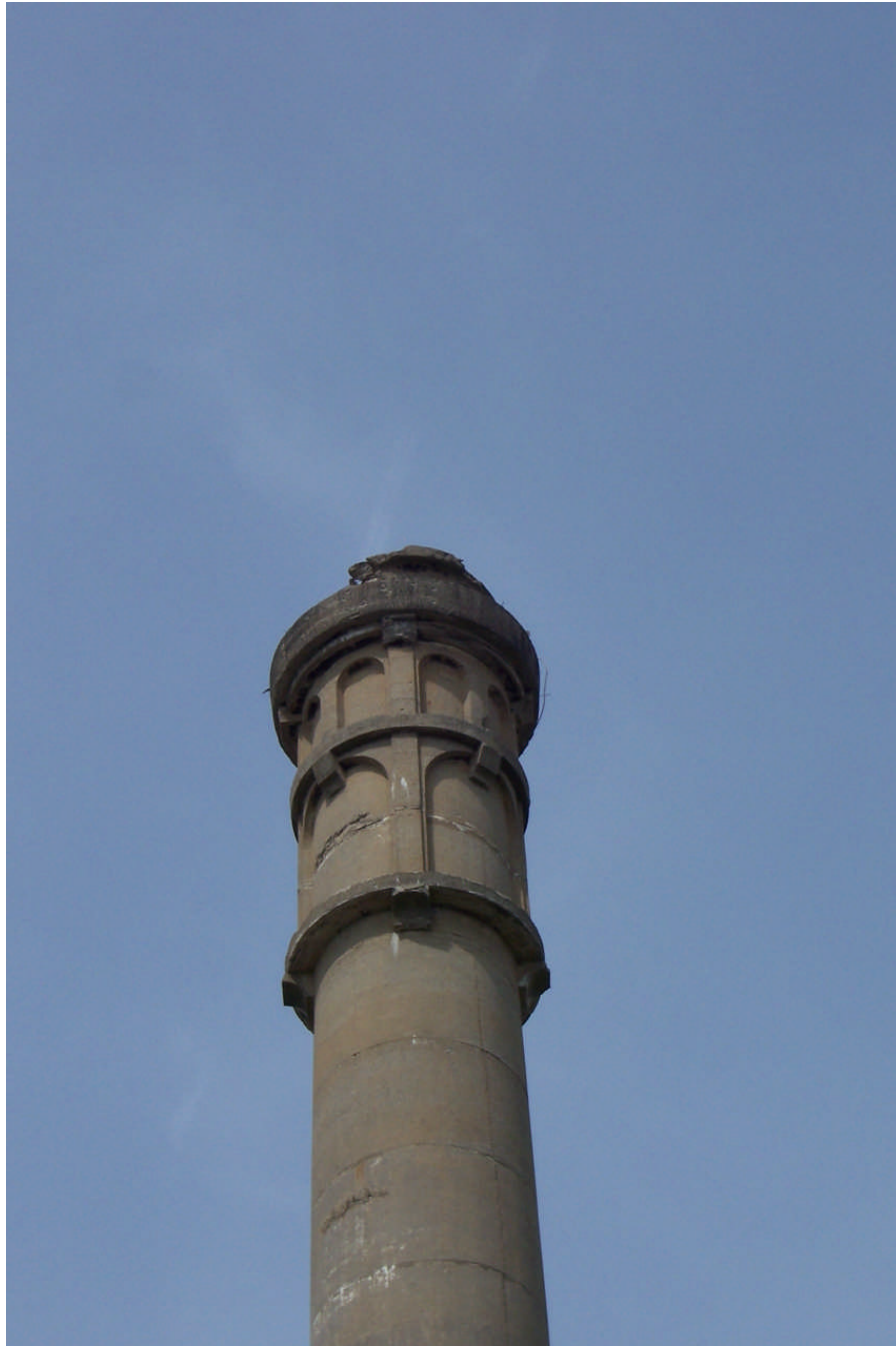
Figure 47. Detail of the top of the concrete smokestack (Building/Feature 6) for the powerhouse. The stack is decorated with arches, banding, and corbels. This smokestack is one of the most ornate documented at a coal mine in Illinois and is indicative of the high-caliber of design employed at the facility (FRR May 2006).
