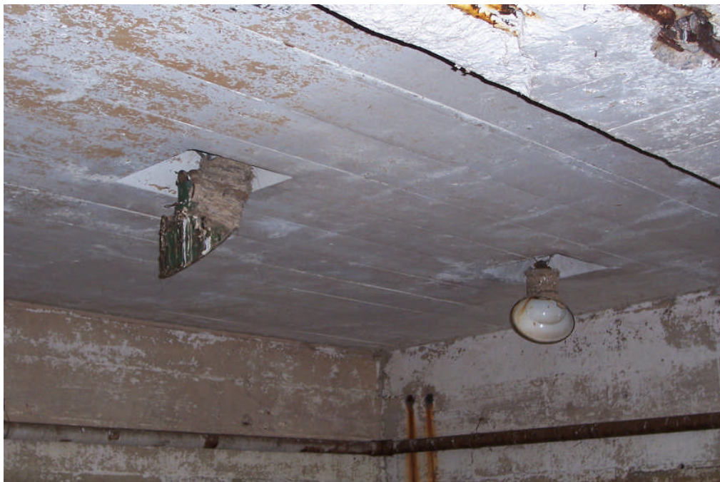
Figure 21. The corridor between Shaft A and the wash house was illuminated by ceiling fixtures spaced 5' to 6' apart and set within niches. Some of the fixtures still remain in place, like these shown above (FRR May 2006).
