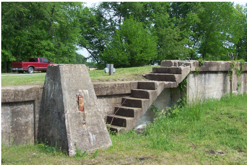
Figure 41. View of the concrete retaining wall running between Shaft A and hoist-engine house. The concrete pier shown formerly supported a steel post or brace for the tibble (FRR May 2006).
